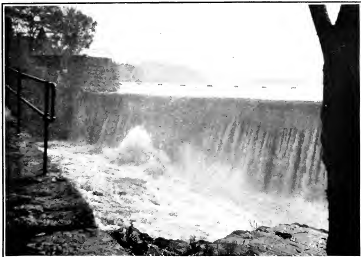
A. HIGH WATER AT LAWRENCE DAM, MERRIMACK RIVER, AUGUST, 1915.
